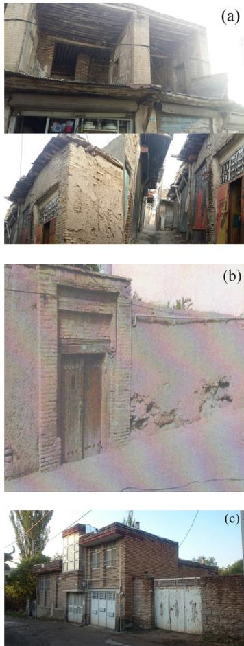
Figure 1. Samples of three categories of masonry buildings in Kermanshah, (a) brick walls with wooden beam, (b) adobe buildings, (c) brick walls with steel beam
