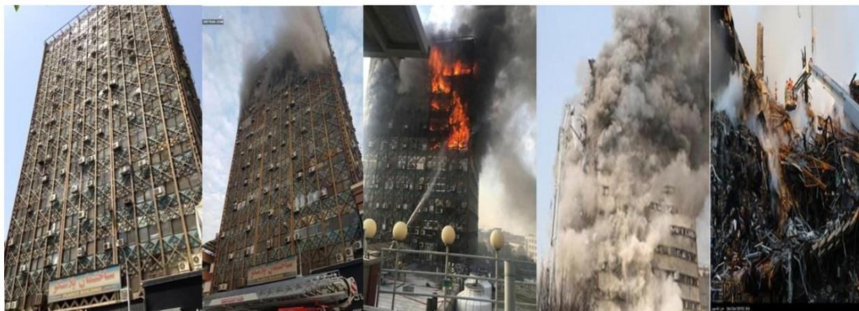
**Fig. 1. The progressive collapse of the PLASCO building in Tehran in 2016 [4].**
